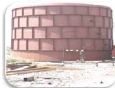
Bunker Shell Fabrication
